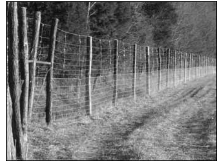
Newly installed 8-foot deer fence.
